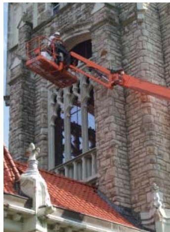
Cranes continue to lift new pieces of stonework into place.
