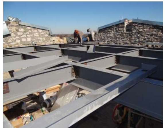
New structural elements have been installed on the roof.
