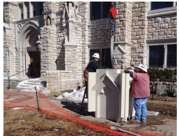
Crews have begun installing pieces of the bell tower.
