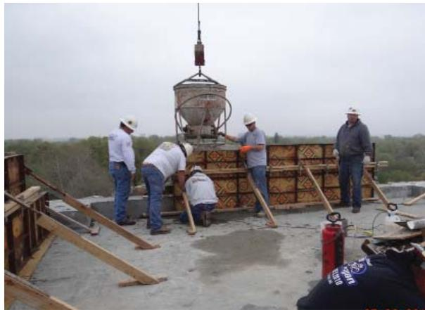
Workers from C & M Construction pour concrete as part of the repair on the bell tower.
