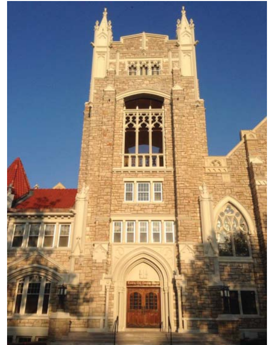
Today with renovation complete
